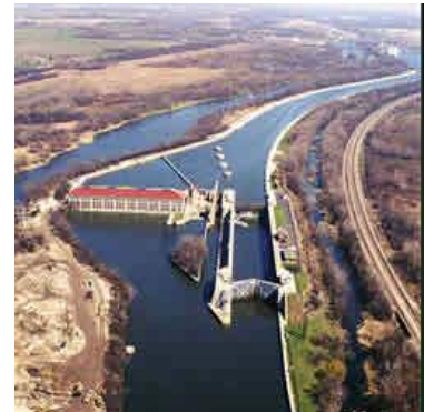
The Lockport Lock on the Sanitary & Ship Canal in Will County, IL, about 35 miles from downtown Chicago.
