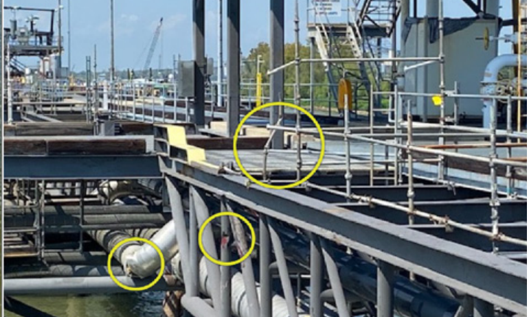
Damage to pier (circled). Left to right: A vertical piling. Insulated pipe, pier support bracings, and railing.
