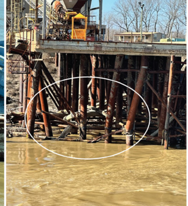
Left to right: The damage to barge ACBL2549 after the contact (circled), and the damage to the Port of West Memphis dock (circled). SOURCE: COAST GUARD.
