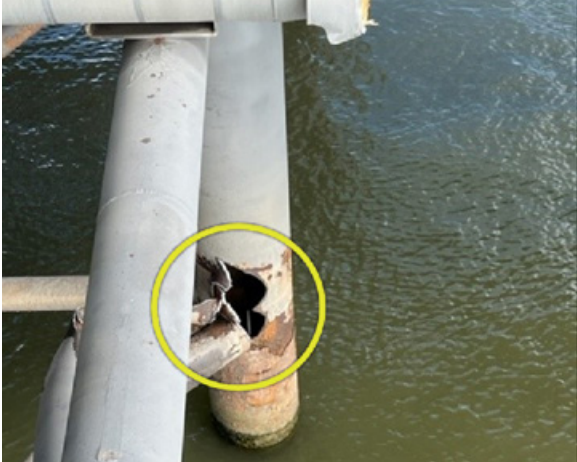
Damage to pier (circled). Left to right: A vertical piling. Insulated pipe, pier support bracings, and railing.
